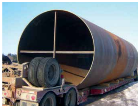
Steel casing being delivered to site
